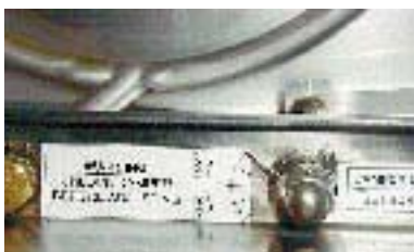
Guillotine or BT damper control damper position indicator and set screw.
