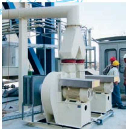
Seal air system
