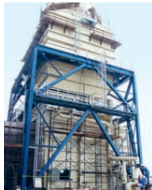
4. Diverter and Guillotine Damper
