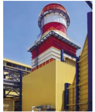
Diverter and Guillotine Damper
