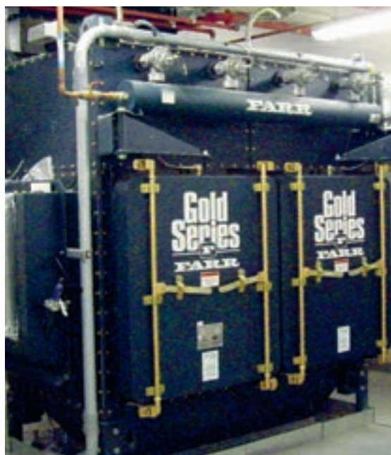
GS8 BIBO on potent compounds from tablet coating
