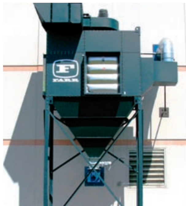
GS20 on aluminium shot blasting
