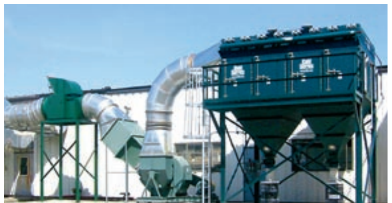
GS48 on wood finish sanding
