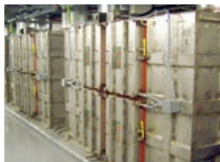
HEPA's after dust collectors
